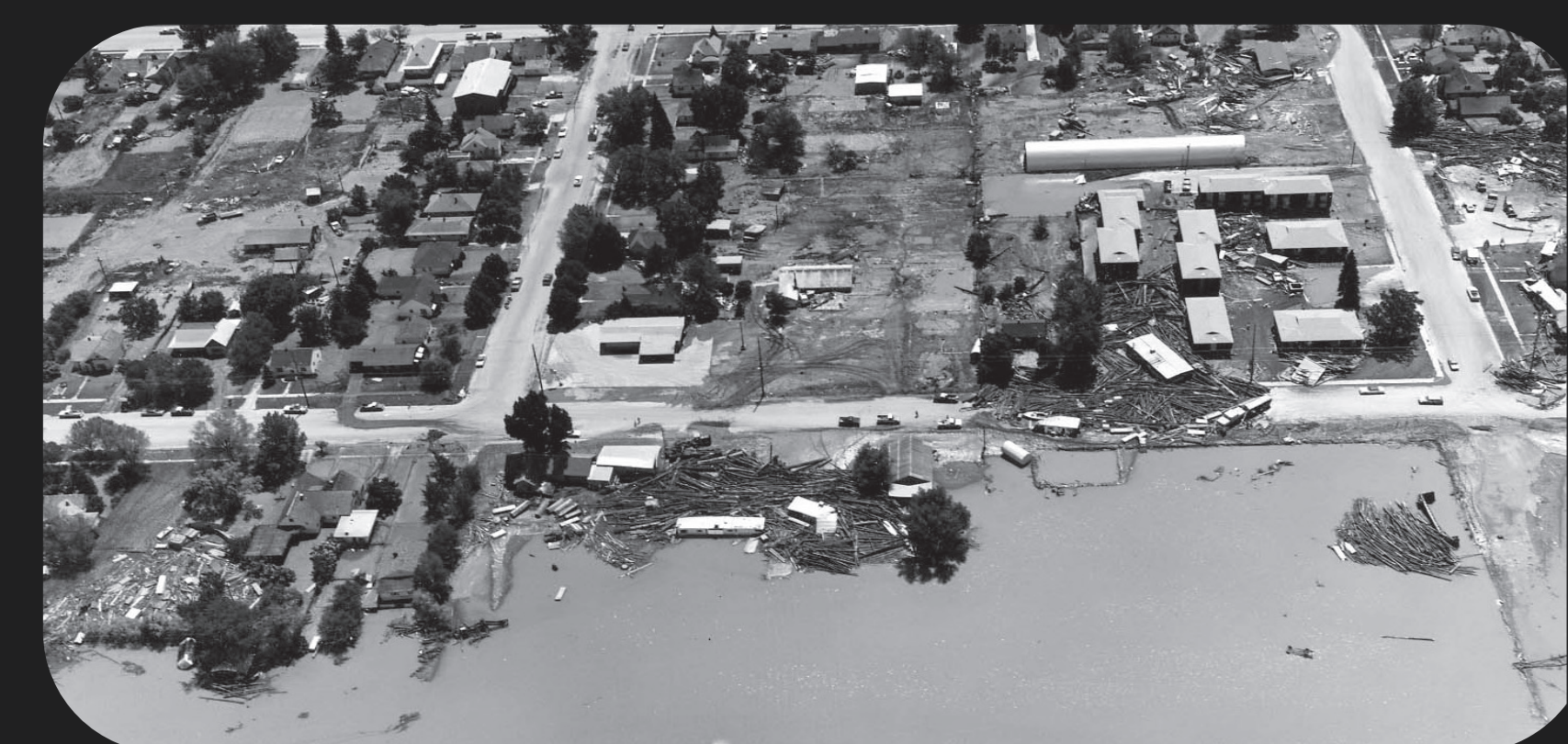
View of Rexburg the day following the breach. There is a house in the middle of the street, and logs from the lumber mill in the foreground are strewn around the area.
